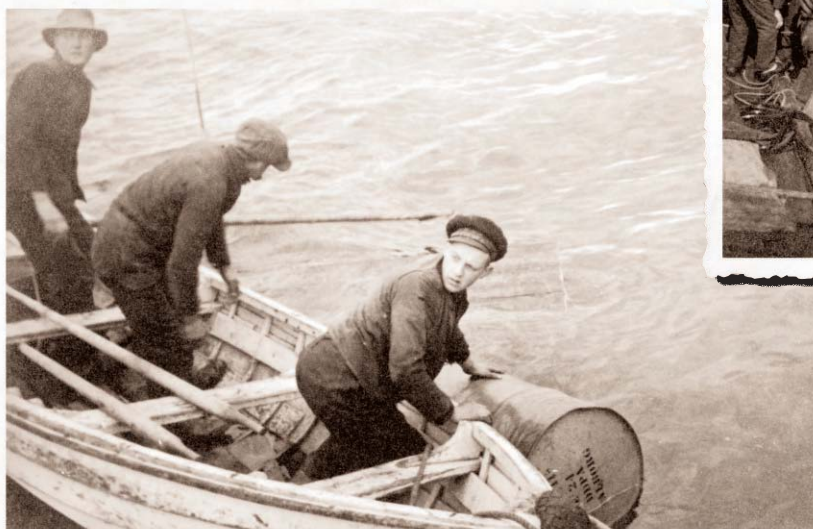
Water-filled oil drums being packed into the hold of M/S Jylland.
