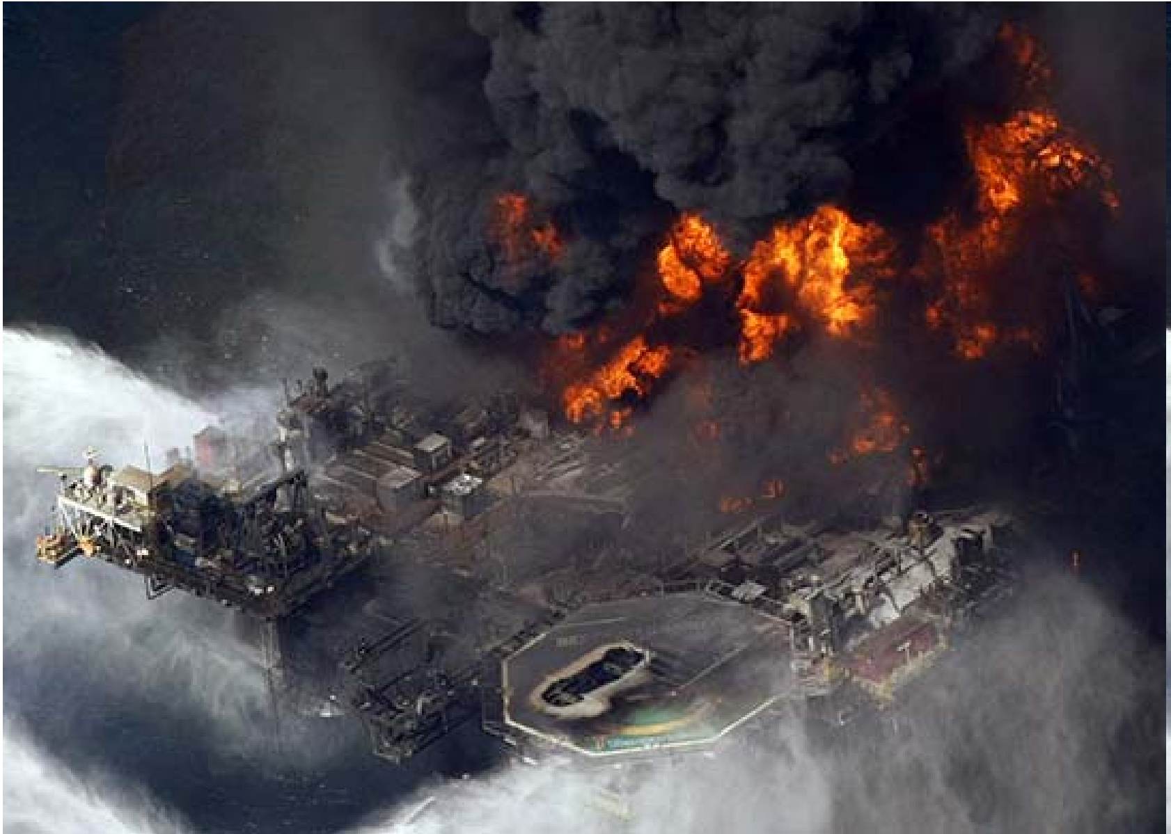
Early morning Day 2 – Note the hole burned through the aluminum helideck
