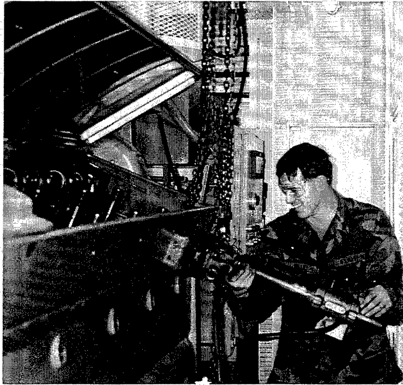
(i) Installing an NG load block.
