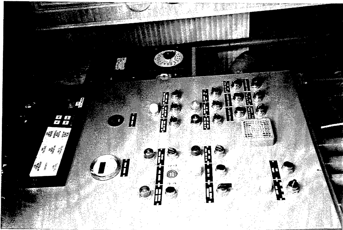
(a) ECP showing status screen (upper right) and gas detect alarm light.
