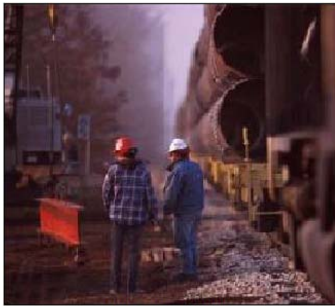
Pipes in Transit
