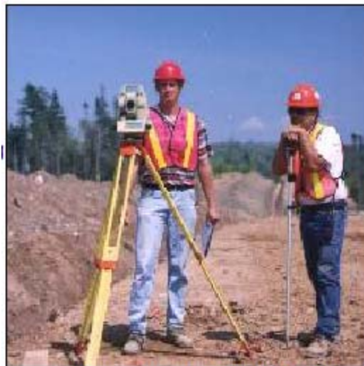
Surveying the Right-of-Way
