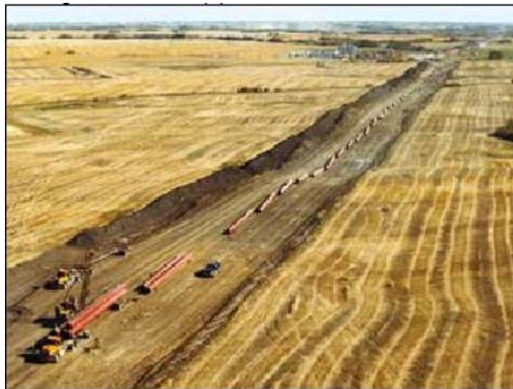
'Stringing' the Pipe
