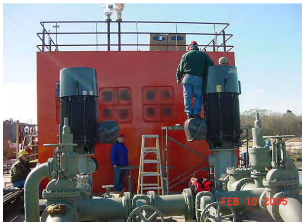
Pumps on a barge
