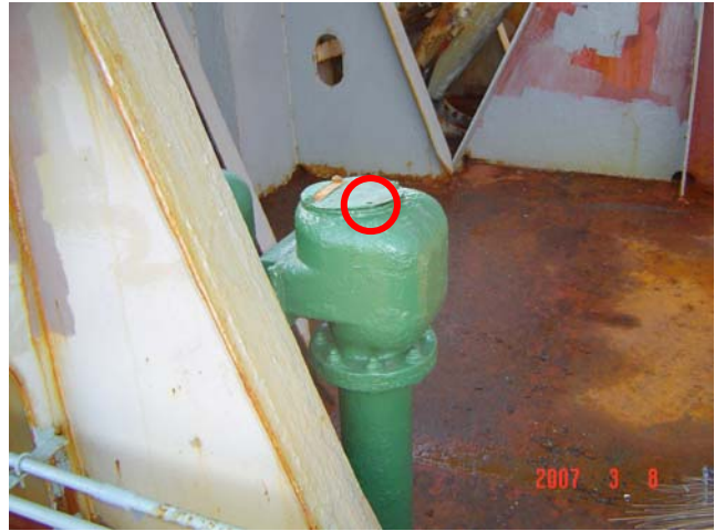
Missing bolt of air pipe head
