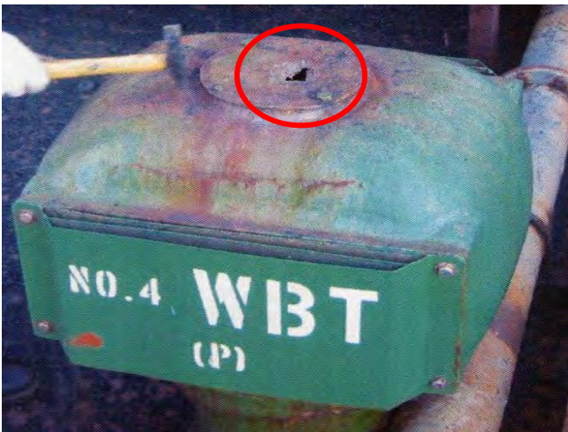
Wastage and holes of air pipe head
