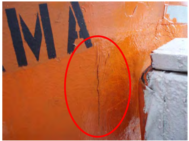
Damage of shell
