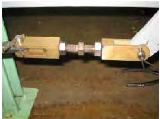
Correct condition of turn buckle
