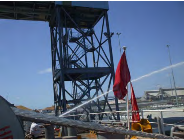
Performance test of emergency fire pump
