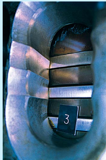
Right: A view of the piston ring area through a scavenging port of a slow-speed engine.
